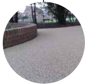
Resin bound gravel surface
